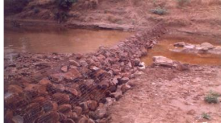
Gabion structure in a stream bed
